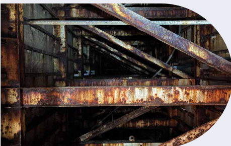
Before application of nC Corrosion Passivator
